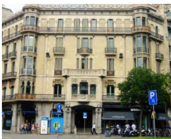
Figure 4-11 A building located in one certain land use might have more than one level and devote them to different activities, multiplying the available area
