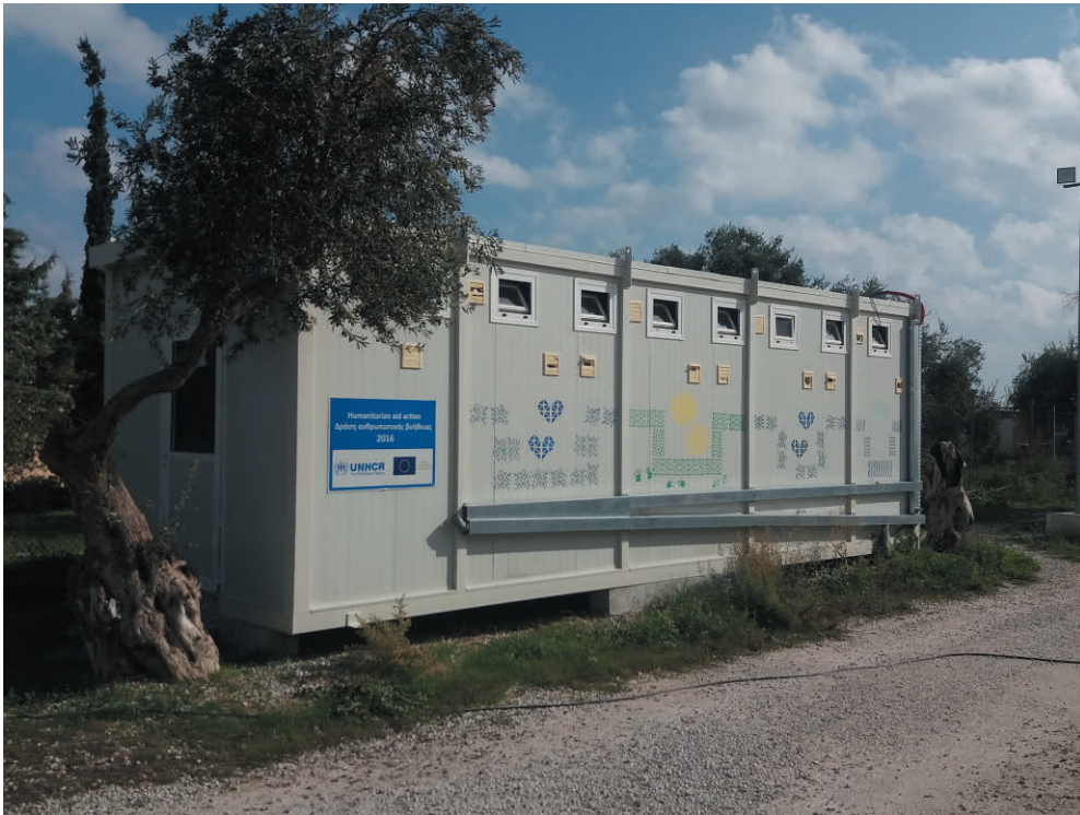
Figure 3.7. Typical building inside the Kara Tepe reception center – this ISO Box container for administration purposes. Photo: Jussi S. Jauhiainen, November, 2019.
